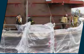
Alternate Access & Scaffolding Solutions
