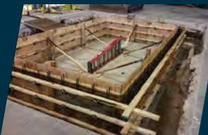
Foundations & Civil Construction
