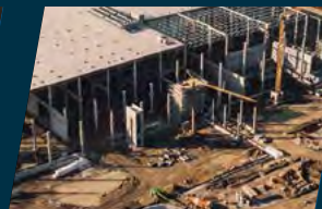
New Build & Plant Relocation
