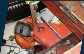
Mechanical Service & Installation
