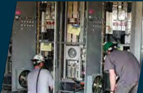
Electrical/Controls Design & Installation
