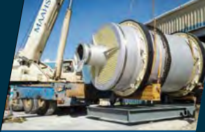
Specialized Rigging & Crane Operators
