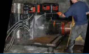
Cleaning, Degreasing, Metalizing & Coatings
