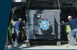
Machine Installs & Specialized Rigging
