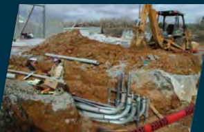
Planning, Surveying, & Site Development
