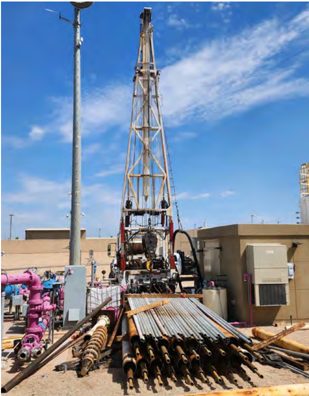
Airlifting with 60T Pump Rig
