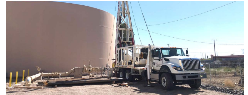
1x 15T Pump Rig
