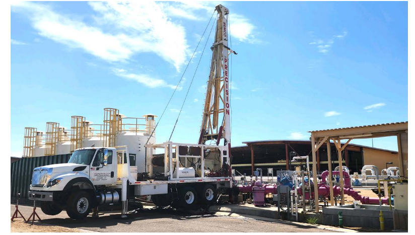
1x 40T Pump Rig
